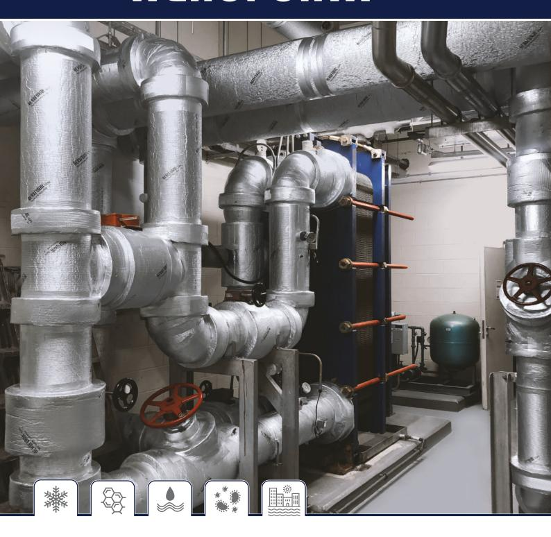
Cross-Linked Closed Cell Polyolefin Thermal Insulation Foam
