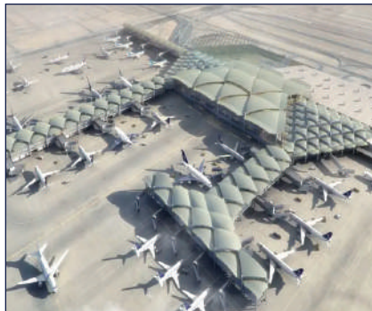
King Khalid International Airport AeroSound® SLM
